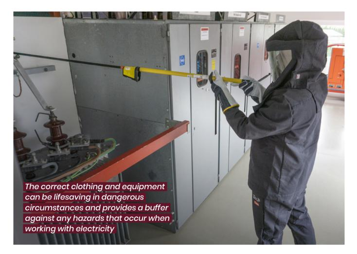
orking in a high voltage (HV) environment should always be approached with the correct personal protective equipment (PPE) and necessary training required to work in or around the high voltage area. It is important to feel confident enough to work around electrical hazards safely, following on from thorough training. To make sure you're as safe as possible when working in a high voltage environment, the following guidance should be remembered and practiced at each HV occurrence.
