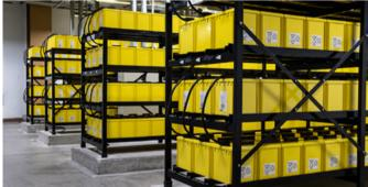
and easy to transport, handle and recycle. Crucially, advanced TPPL technology significantly improves energy efficiency, by providing up to 43% energy reduction compared with traditional VRLA batteries through reducing float current requirements. Further energy savings accrue as it can operate, within warranty, at elevated temperatures, reducing air-conditioning requirements.
