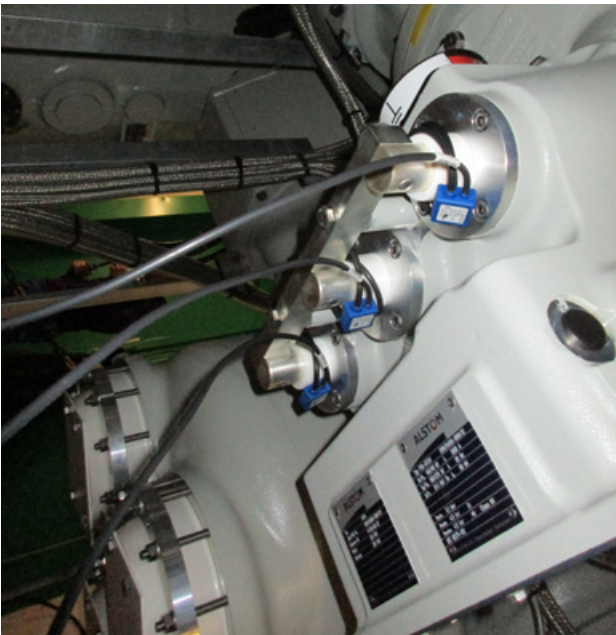
Figure 3: Rogowski coil connection on an earthing switch
