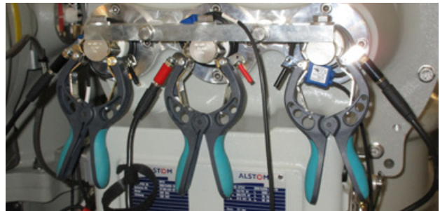
Figure 4: Current injection and Rogowski coil connection on an earthing switch
