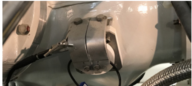
Figure 5: Current injection and Rogowski coil connection on an earthing switch
